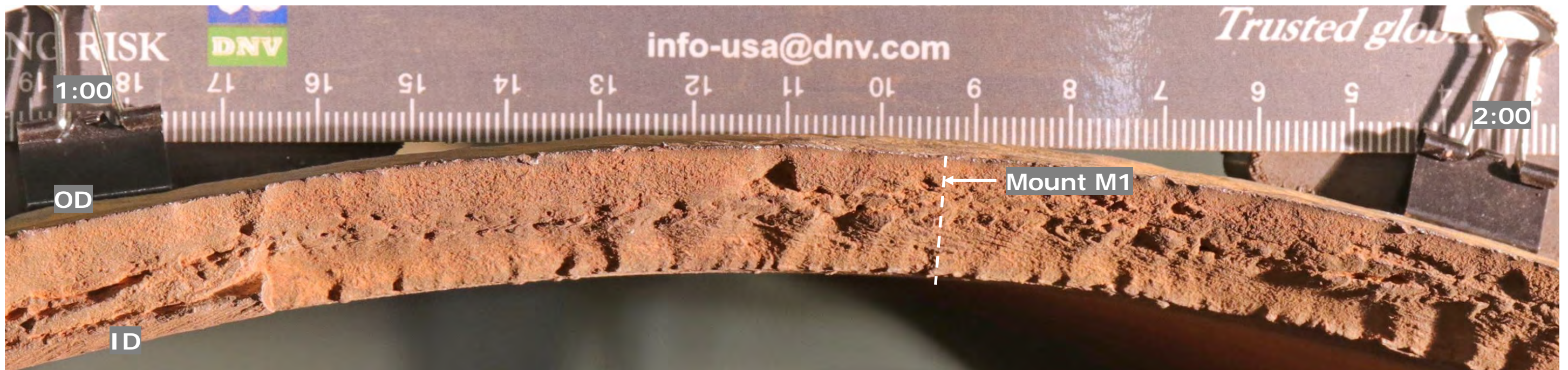
Figure 21. Photograph of the fracture surface of PS A between the 1 and 2 o'clock orientations. Units of ruler are in cm. Flow direction is into the photograph.
