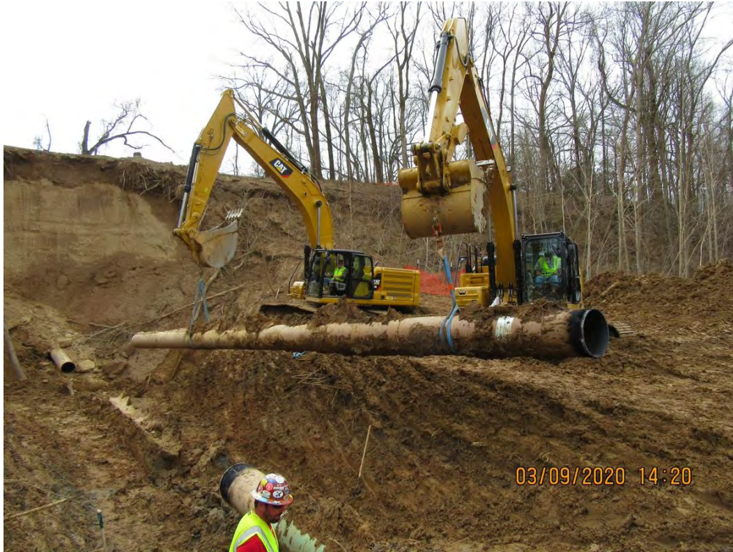
Figure 9. Upstream Pipe Section During Removal
