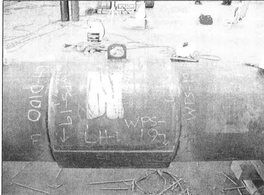
Figure 3. In-service tight-fitting repair sleeve.
