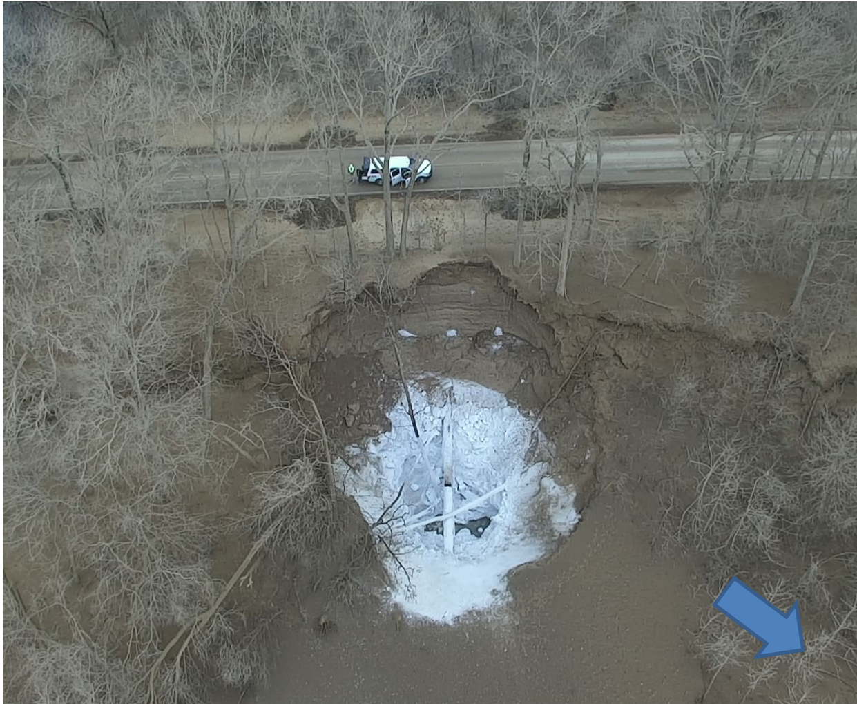
Figure 2: Vehicle is Parked on HWY 433 - The White is Ice Generated by the Release of CO 2 - The Blue Arrow Points North (Aerial Drone Photograph Courtesy of the Mississippi Emergency Management Agency)
