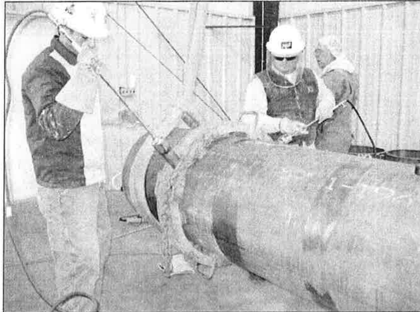
Figure 1. Typical setup for girth weld procedure qualification.
