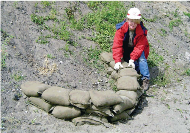
Corps employees demonstrate building a ring dike.
