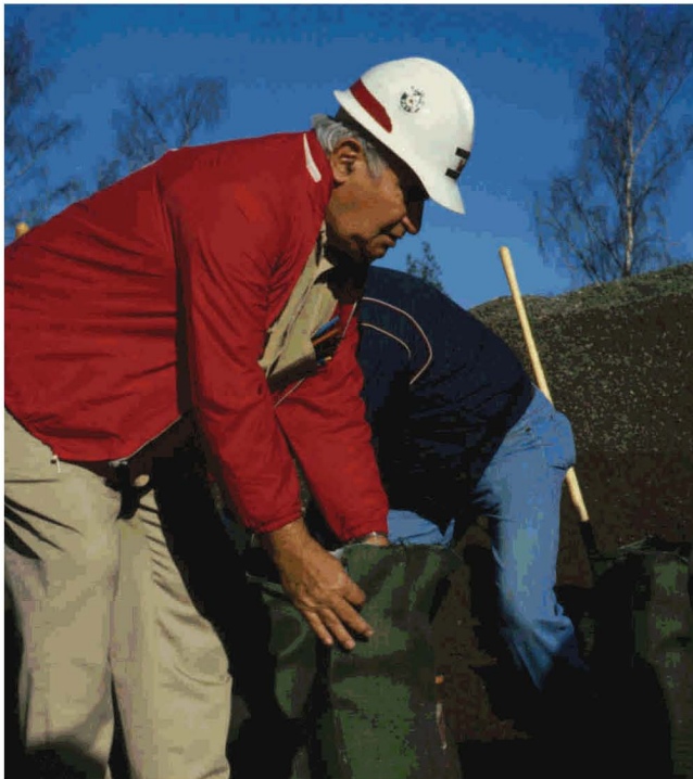
Veteran flood engineer Ernie Sabo demonstrates that the sandbag should be two-thirds full, folded at the top.
