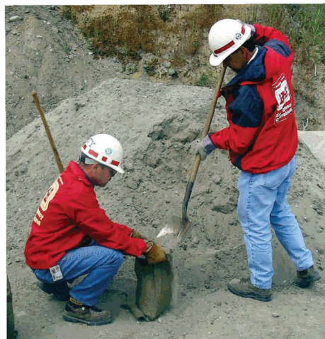
This two-member team uses correct positions for sandbag filling.
